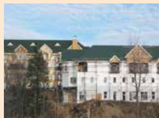
Centre de santé SPA Bromont Bromont Commercial building
